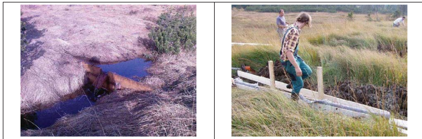
Fig. 33 Constructed check dams at Klugeho louka
