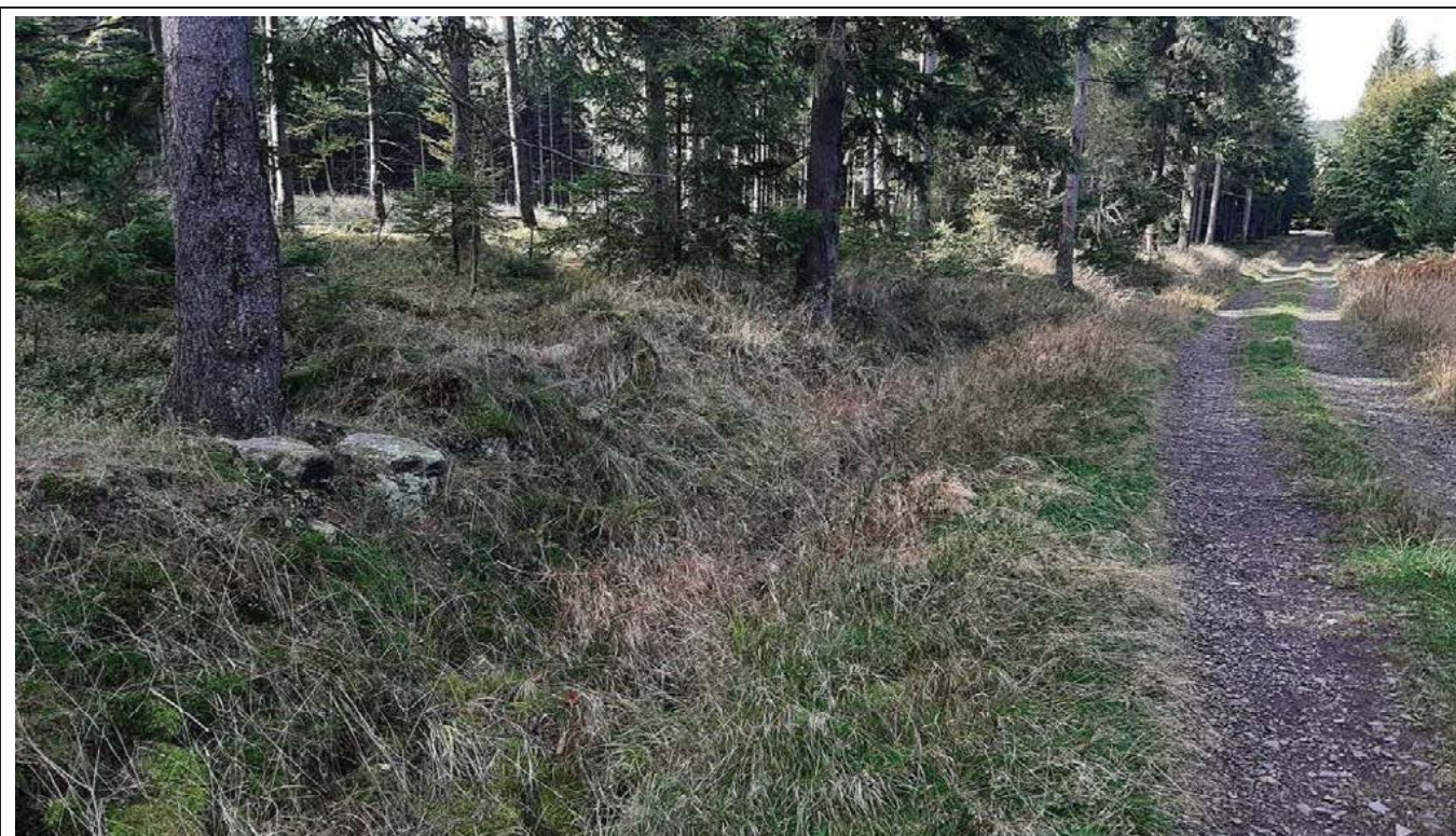
Photo 8 Ditch along the road without culverts at site 6 Water divide Hlava – Jordán
