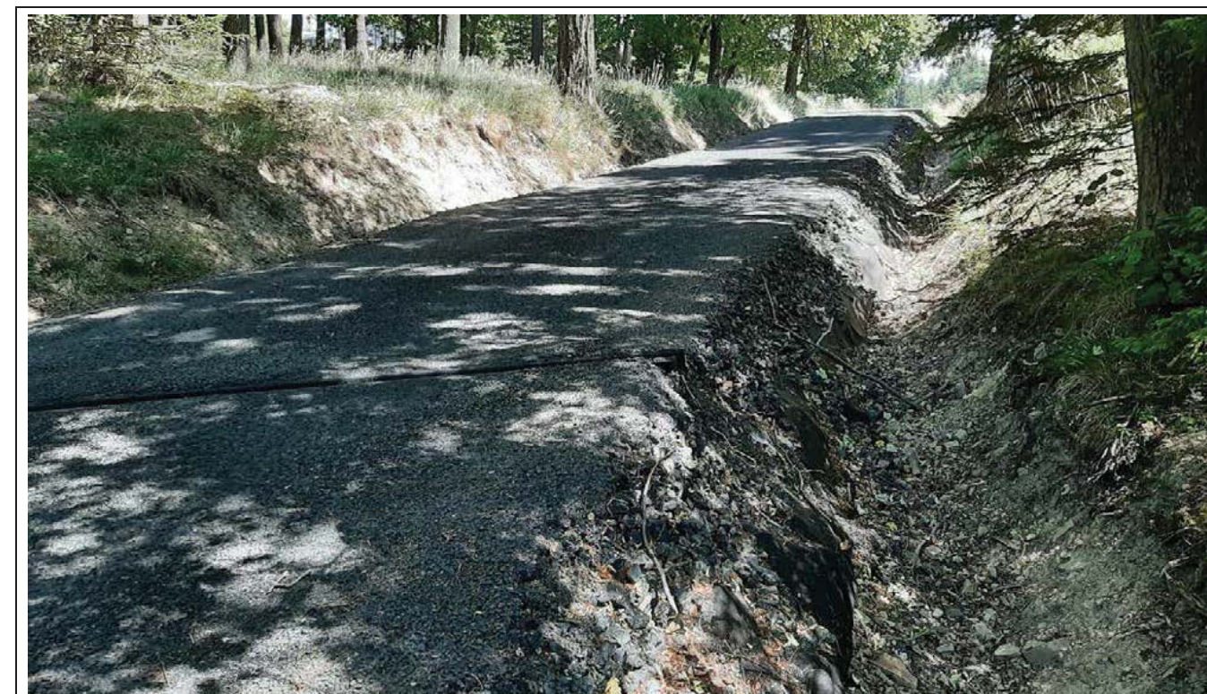
Photo 11 Example of unsuitable drainage of the road – site 3 Spring area of the Třítrubecký potok Brook
