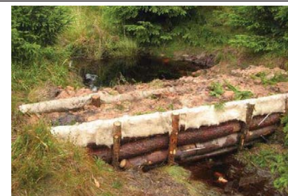
Fig. 25 Double sealed log dam
