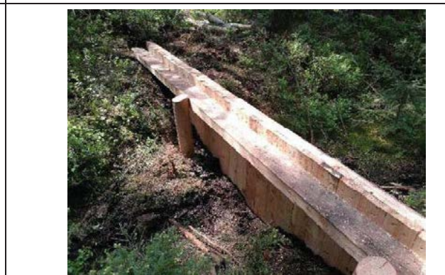
Fig. 30 Constructed check dams
