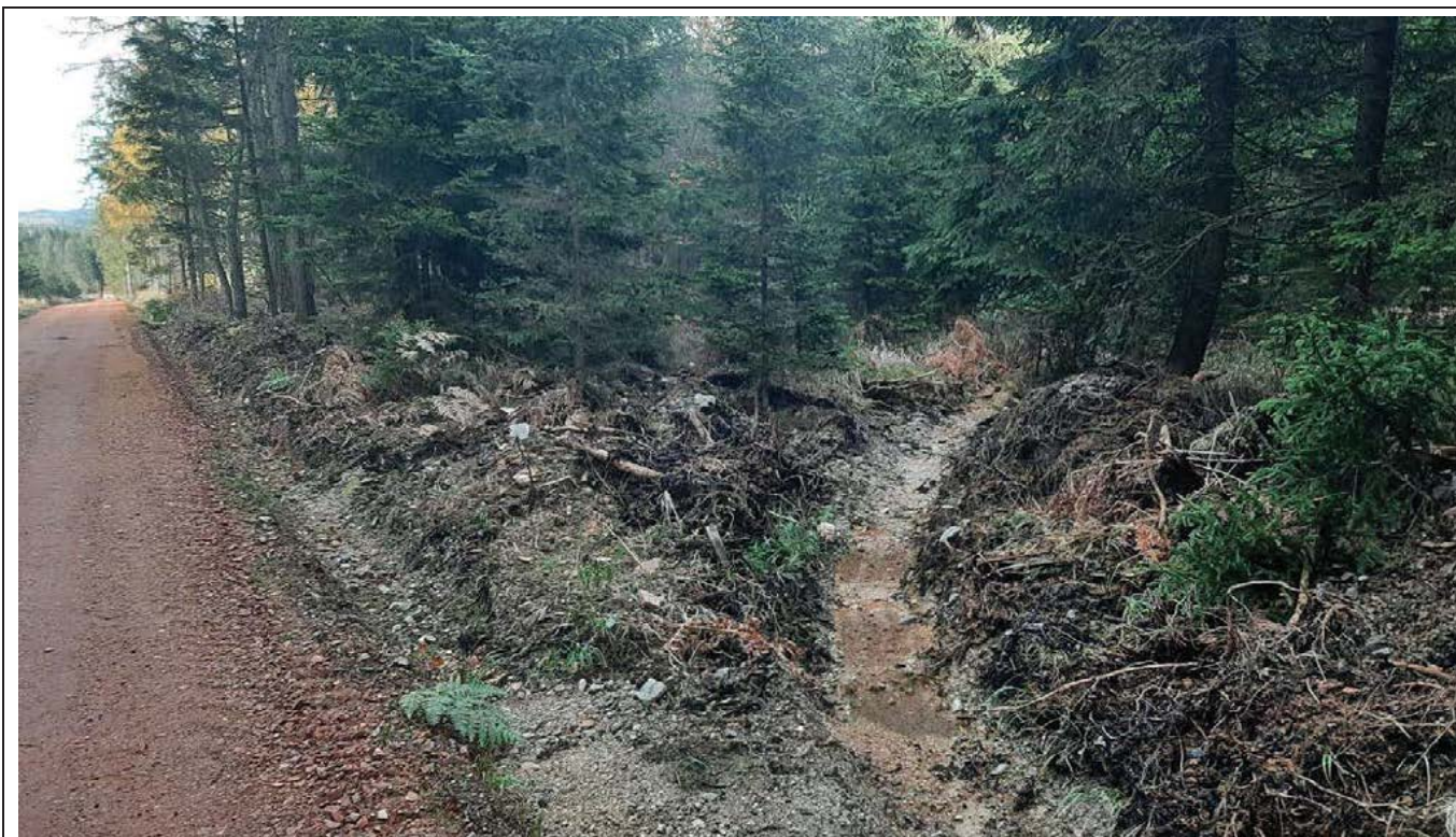
Photo 12 Demonstration of the road ditch relief at site 1 Voložný potok Brook
